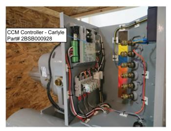
Fig. 30 — CCM Mounted inside Compressor Box
